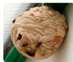
Secondary nest in a building.
